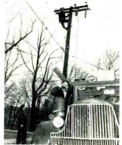
UTILITIES are tied in
