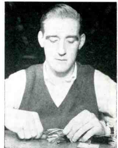
FIG. 2—Old method of removing shields involved snipping with shears. New methods are shown in Fig. 3 and 4
