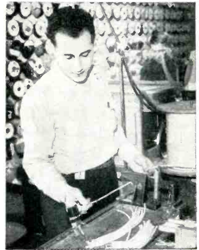
FIG. 1—Setup for cutting uniform wire lengths. Shear jaws are actuated when wire end comes in contact with switch
